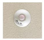
Figure 9- Typical Remote Mounted Lighting Occupancy Sensor
